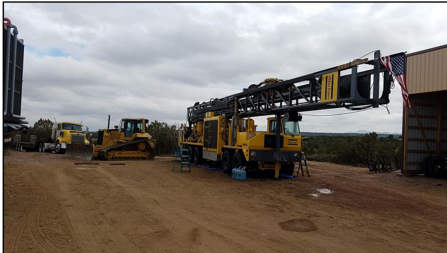
Figures 1&2: Atlas Copco RD20 - Range 3 Drill Rig Being Serviced in Preparation for Drilling of the Amerigo Vespucci # 1 Well
