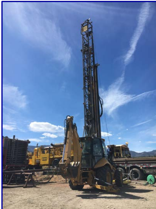
Drilling Operations Progressing well on the Columbus #1 well
