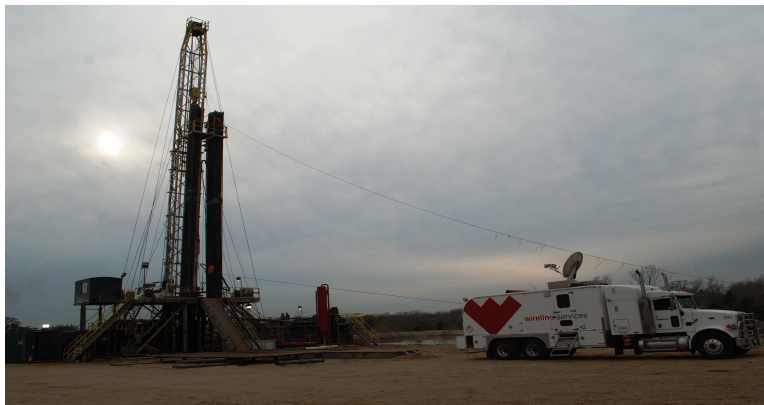
Weatherford on-site site running E-Logs
